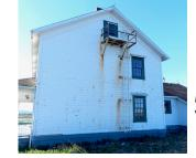
Metal corrosion / wall staining
