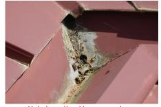
Hole in gutter / improper slope
