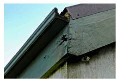
Missing gutter end cap / deteriorated fascia
