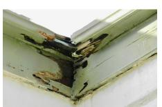
Wall staining and spalling stucco
