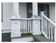
Columns, bases and railing deteriorated
