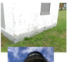
Stucco spalling/ poor drainage away from building
