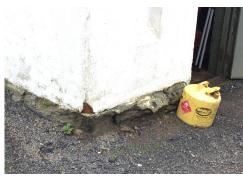
Deteriorated foundation / combustibles in building
