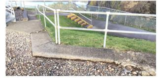
Sidewalk cracks and heaving
