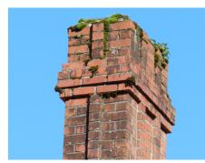
Organic matter on chimney/deteriorated brick
