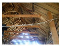
Plates temporarily held in place with steel cables with turnbuckles
